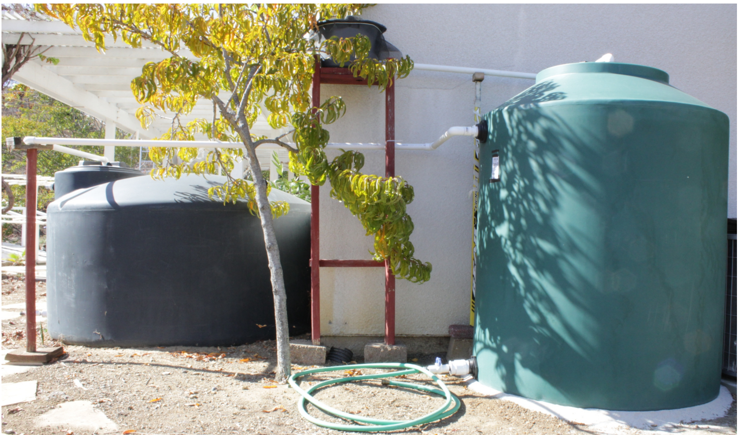
Water pipe connection of 550 gallon rainwater tank (Left) and 350 gallon rainwater tank (Right)
