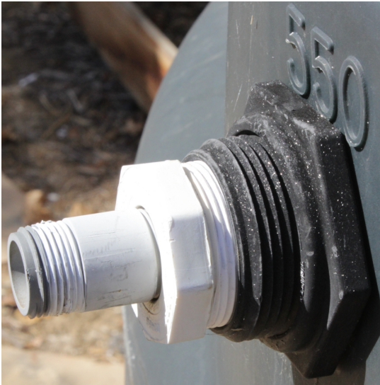
Overflow outlet with garden hose nipple
