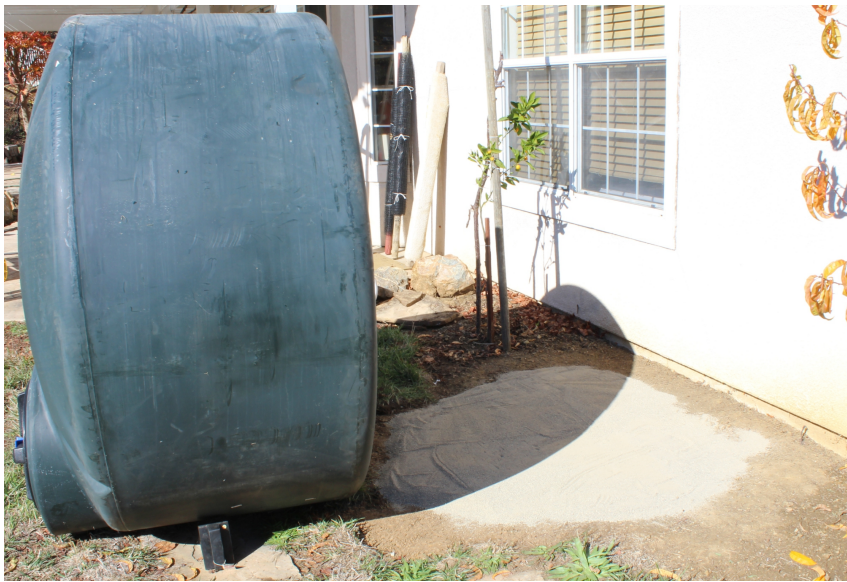
Flatten Foundation with Sand Bed
