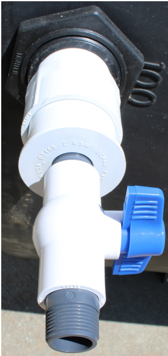
Couplings of lower drain to connect garden hose (Tentative connection)
