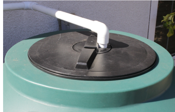
Rain water inlet pipe connection
