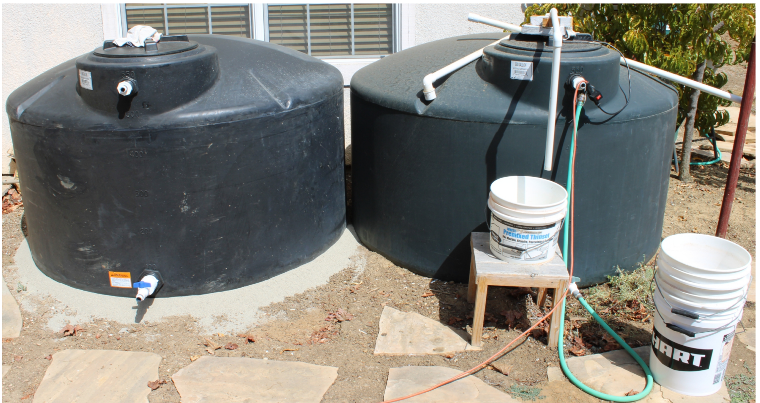
Additional 550 gallon tank newly placed (Left) Old 550 gallon tank in actual use (Right)
