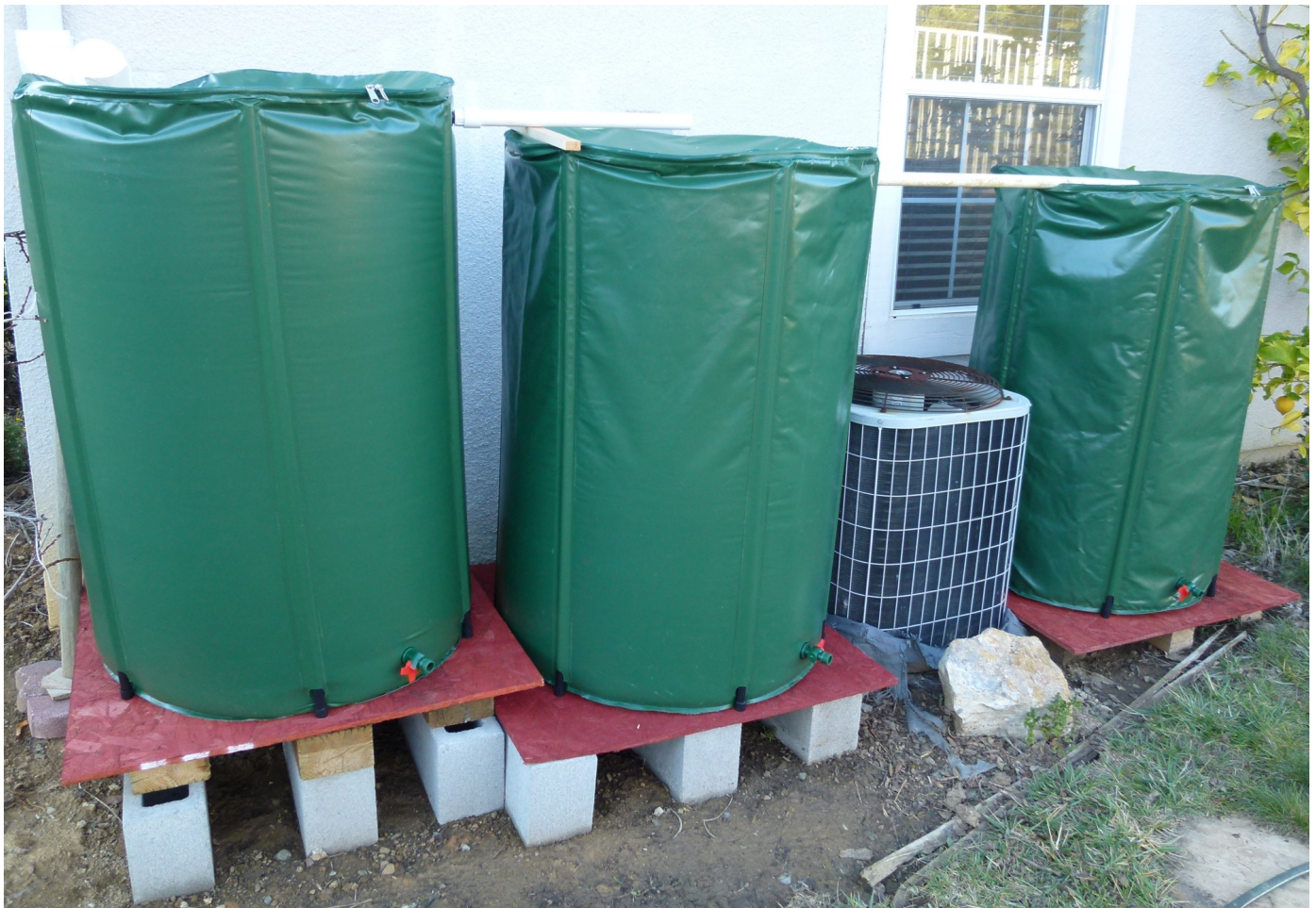
Three Tanks Serially Connected (Total 468 Gallon)
