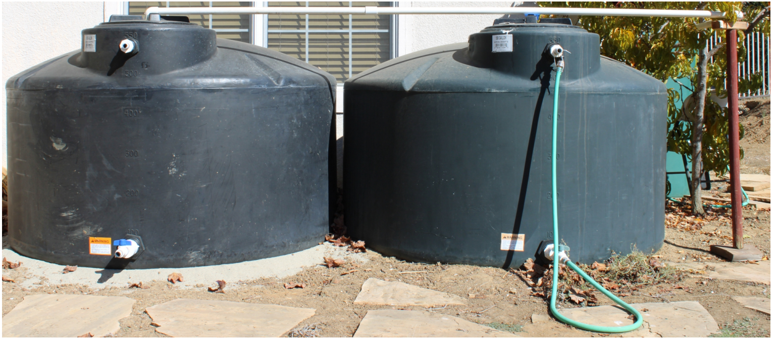
Newly installed 550 gallon tank (Left) ready to store rain water bypassing old 550 gallon tank (Right)
