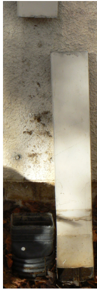
Rain Gutter Cut out
