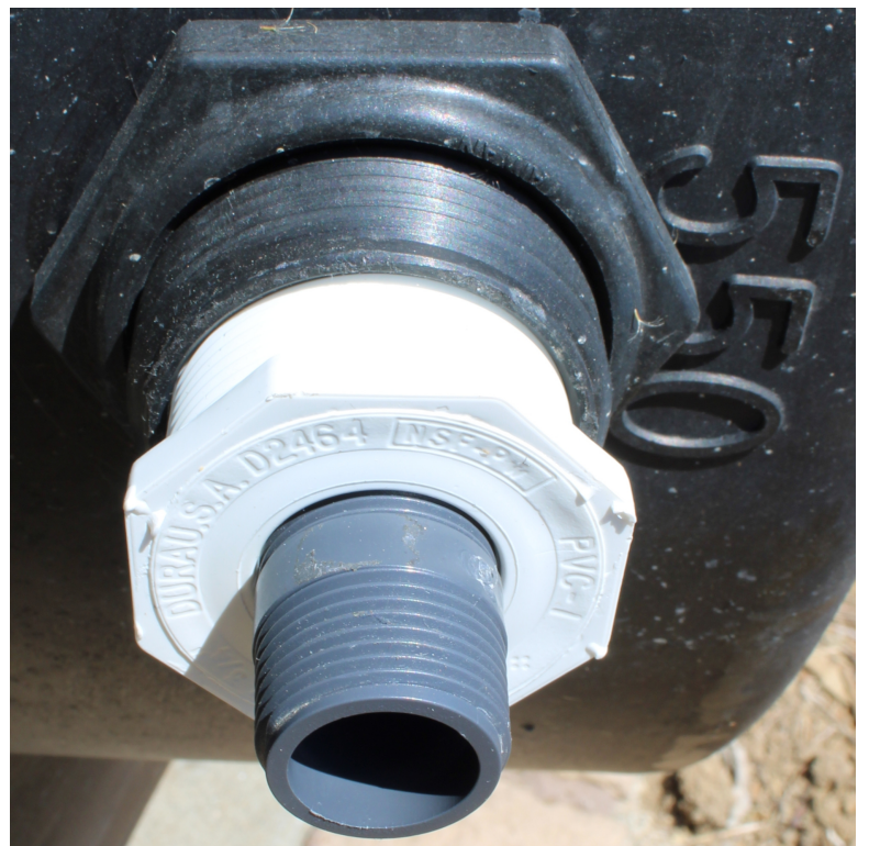
Couplings for overflow drain to connect garden hose (Tentative connection)
