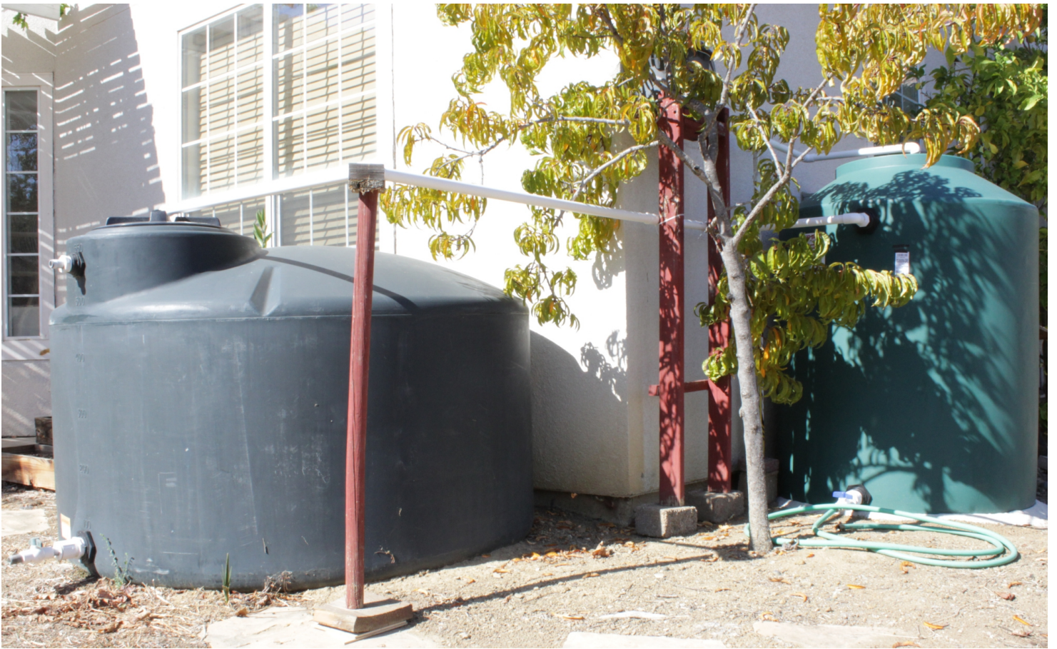
550 gallon rainwater tank gets overflowed water from 350 gallon rainwater tank
