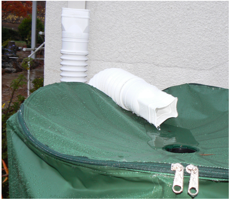
Flexible Downspout Extension to Tank Inlet
