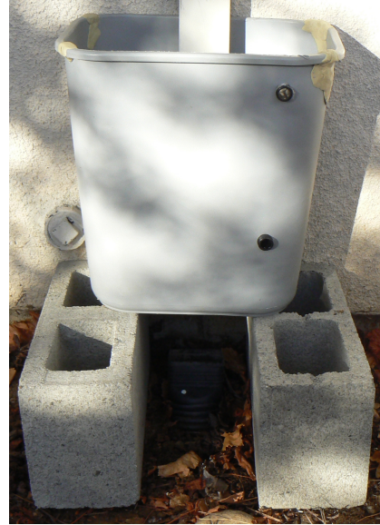
Water Tank (Buffer) Raised by 8" (H) Concrete Blocks
