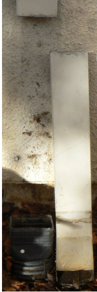
Rain Gutter Cut out
