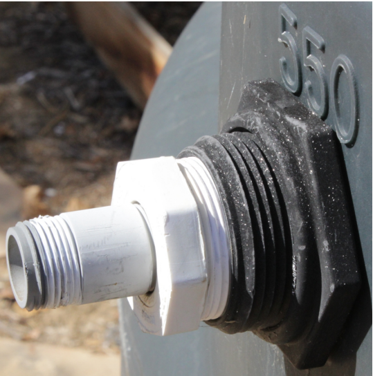
Overflow outlet with garden hose nipple
