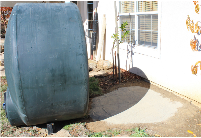
Flatten Foundation with Sand Bed
