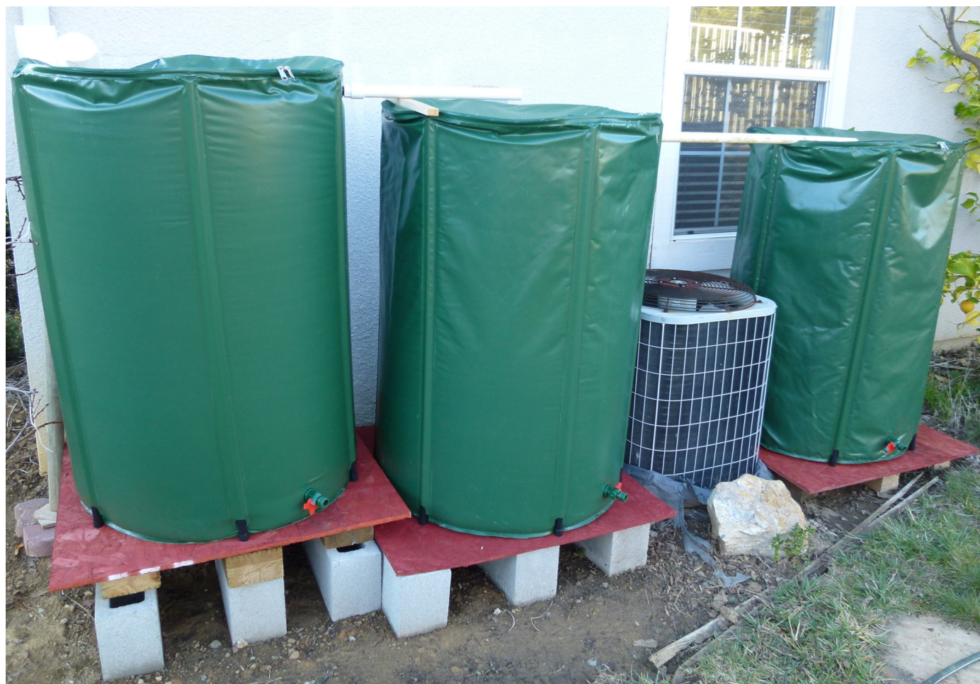
Three Tanks Serially Connected (Total 468 Gallon)
