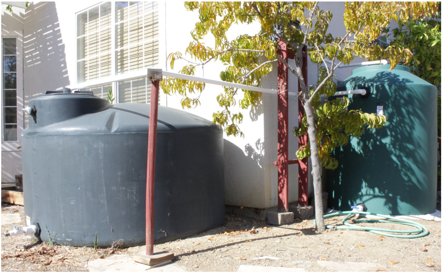
550 gallon rain water tank gets overflowed water from 300 gallon rain water tank
