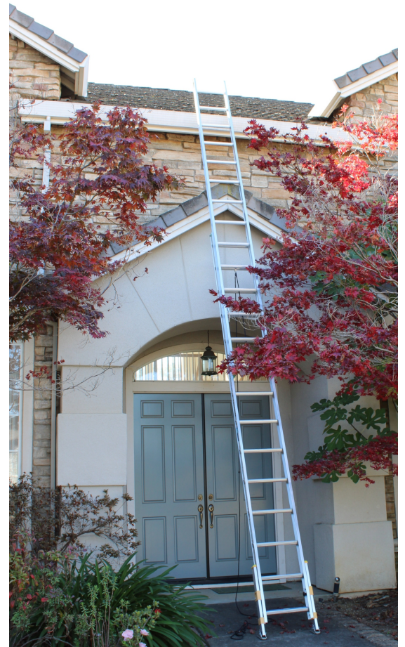
16' long gutter of two story house
