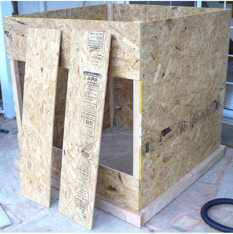
Frame Assembled with 4 Segmented Front Boards
