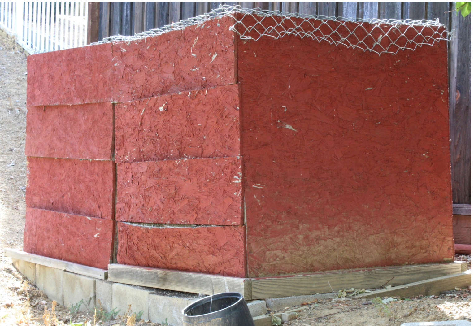
One More Box Added, Painted, & Galvanized Steel Chain Link Roof to Protect from Animals' Intrusion
