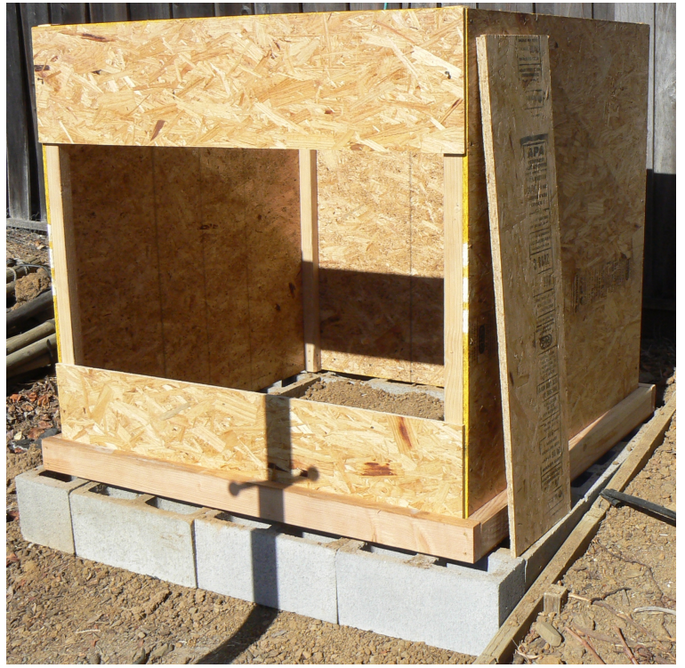
Located on Concrete Block Basement
