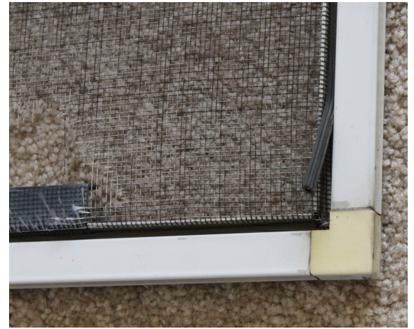
Start from here (Pull up Spline at End)
