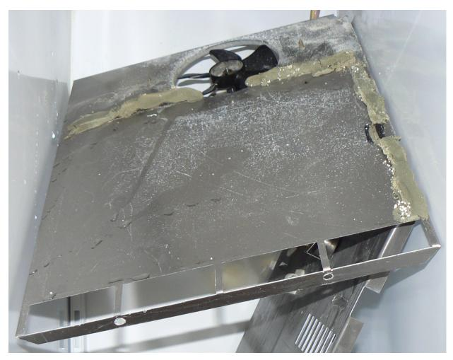
Putty Placed on Metal Board (Partition between Evaporator and Freezer Compartment) Cooling Fan Attached
