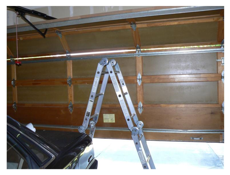
Garage door keeps opening steadily balancing heavy door weight (downward) & hoist energy (upward) generated by torsion spring. Garage door opener (Electric motor) generates smaller power to SHIFT the door up and down.
