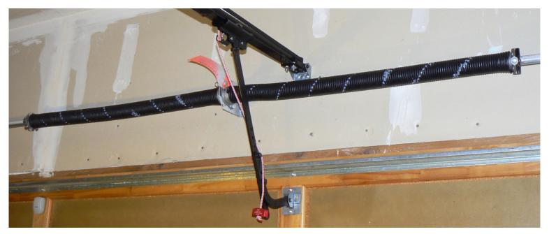
New Torsion Spring Mounted & Winded
