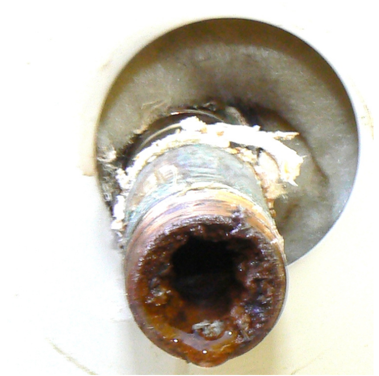
Flush Drain Hole
