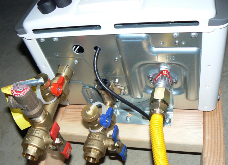
Tankless Water Heater Connection (Tentative)
