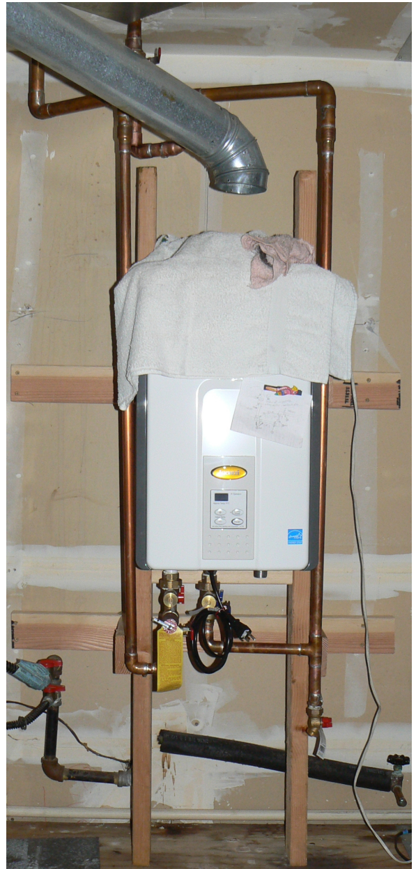
Copper Pipe Routed & Connected
