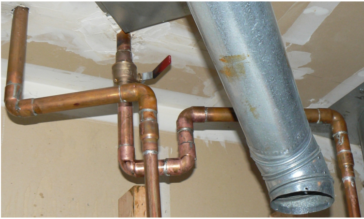
1" Water Shut off Valve Replaced
