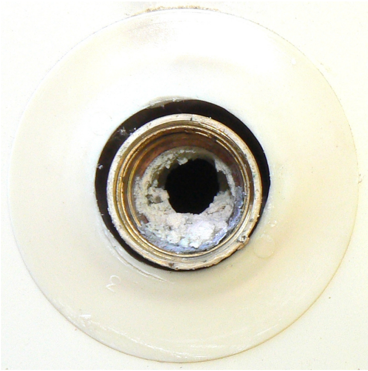
Pressure Release Valve Hole
