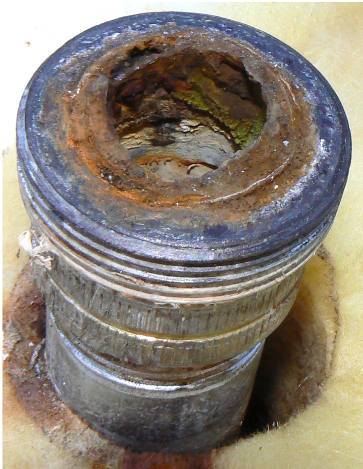
Water Outlet Hole
