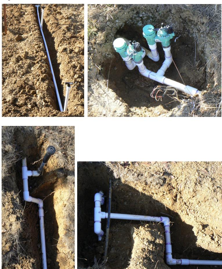
1" PVC piping for water drip line at sloping ground needs a certain special pipe fitting technique.
