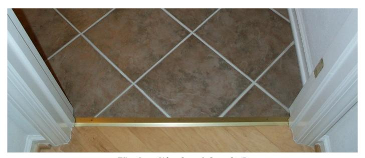
Tiling Done (After Grout & Grout Seal)
