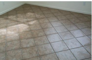
Tiles Glued to Floor by Tile Adhesive (Before Grout)
