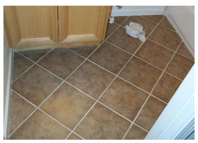
Tiling Done (After Grout & Grout Seal)
