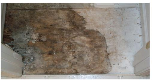
Water Leak Found after Removing Vinyl Flooring
