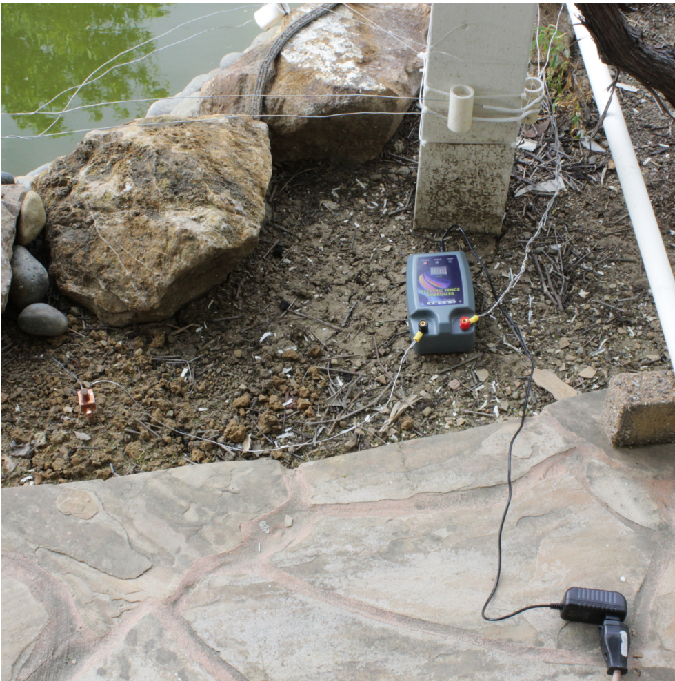
Tentative connection (Ground to both earth rod & pond water)
