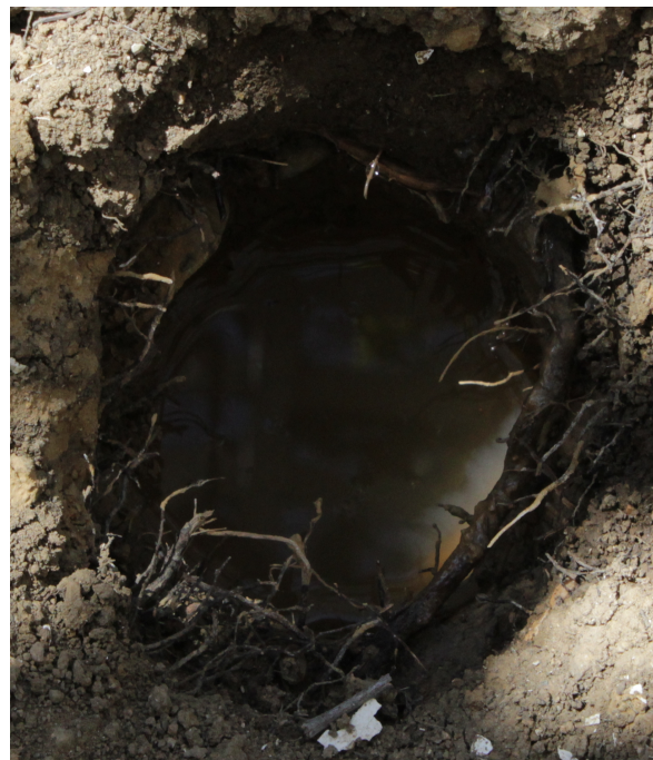
Hole dug down for installing earth rod
