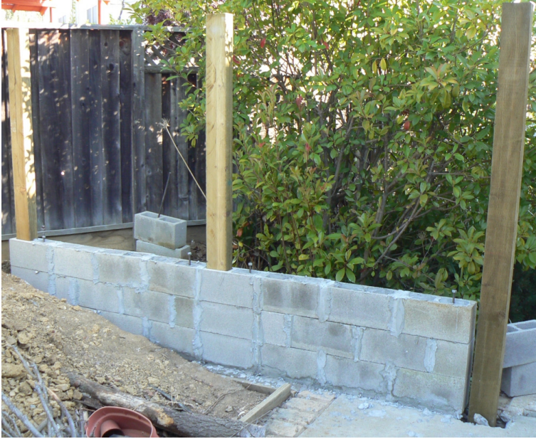
Three Stacked Concrete Blocks with Anchor Bolts
