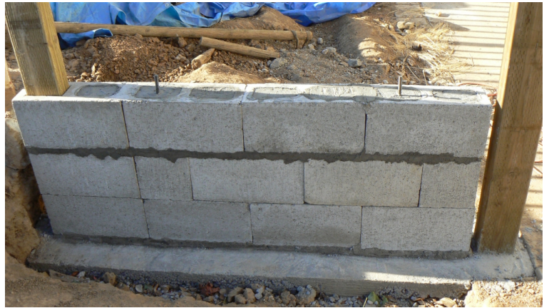
Three Stacked Concrete Blocks with Anchor Bolts
