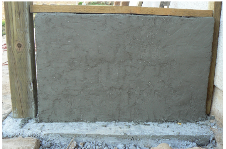
Bonding Cement with Fiber
