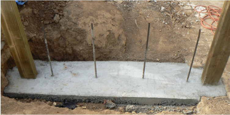
Foundation for Rebars & Pillars
