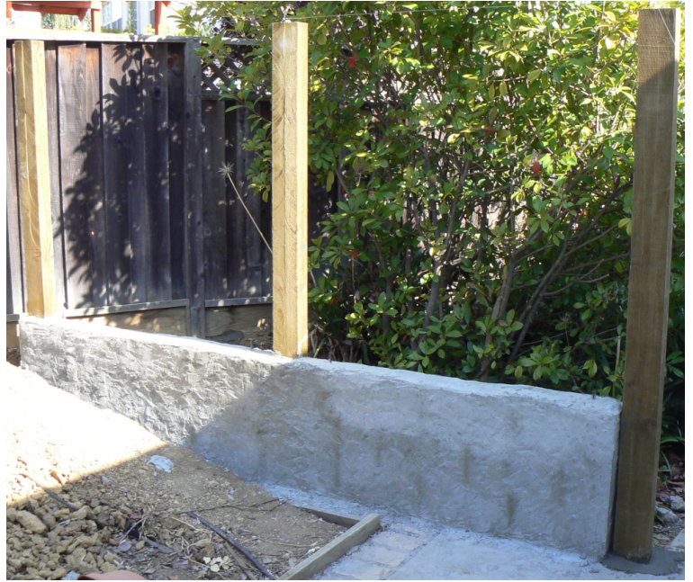
Bonding Cement with Fiber
