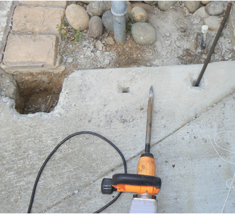
Demolition Hammer for Making Holes and Space
