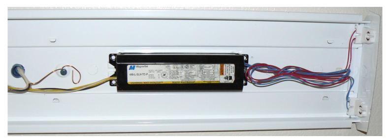
Original Wiring for Fluorescent Tube Housing (Right Portion)
