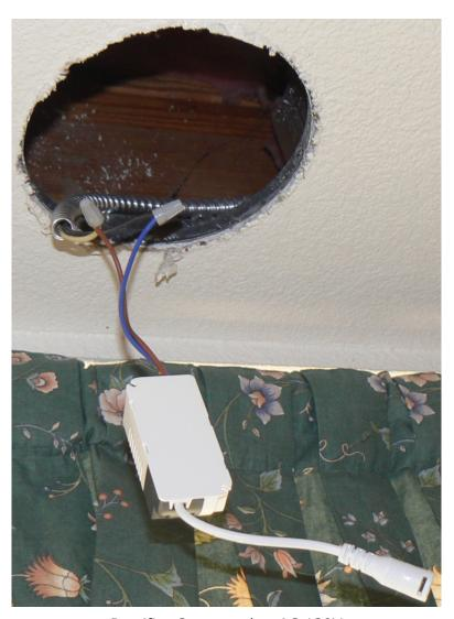
Rectifier Connected to AC 120V
