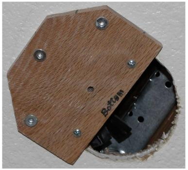
Boards Attached to Ceiling Board
