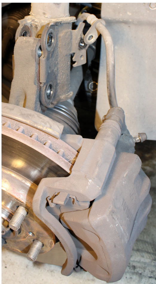
Nuts and bolts removed without detaching brake caliper
